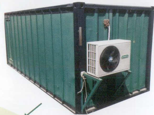
CONTAINER 2 WITHOUT ROCKWOOL INSULATION
